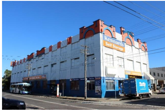
Figure 24: View of front and side of building, south west aspect
