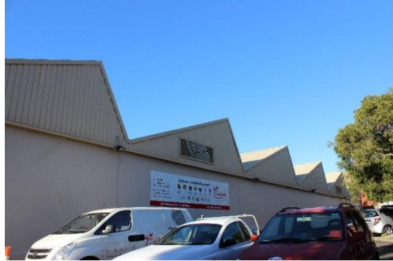
Figure 12: View of façade on Shepherd Street, south east aspect
