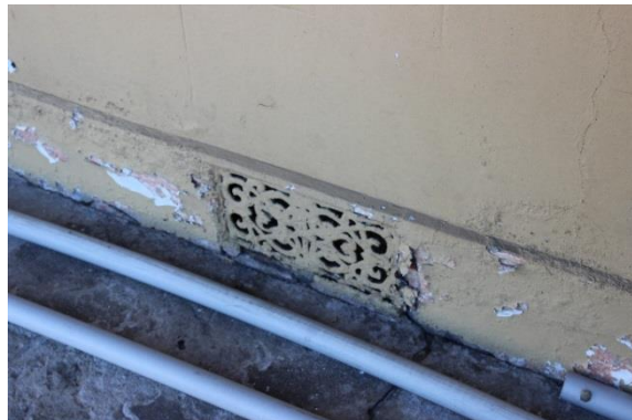
Figure 41: View of iron underfloor vent, west aspect
