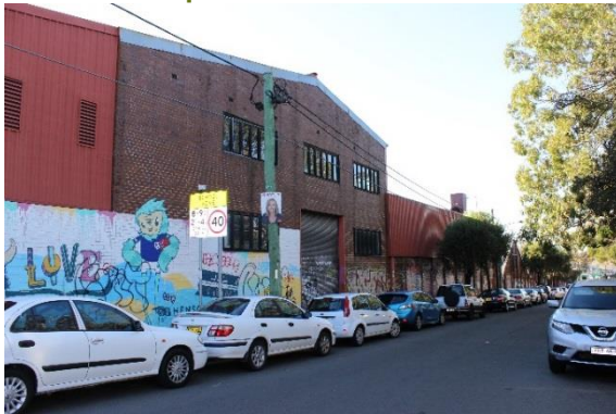
Figure 15: View of façade on Chapel Street, north east aspect
