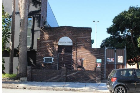
Figure 22: View of building, east aspect
