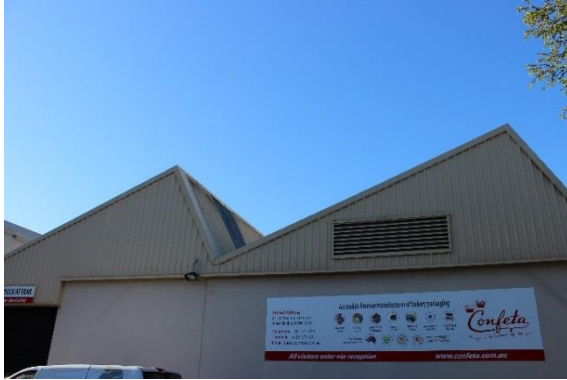
Figure 11: View of roof detail on Shepherd Street, east aspect
