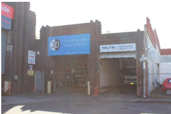
Figure 27: View of façade on Hans Place, north aspect
