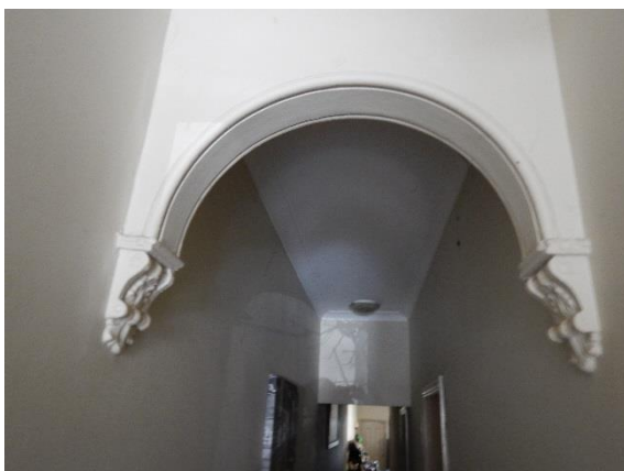
Figure 64: View of original pedestal arch with mouldings in cottage 29
