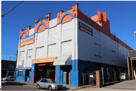
Figure 23: View of side of building on Chapel Street, south aspect
