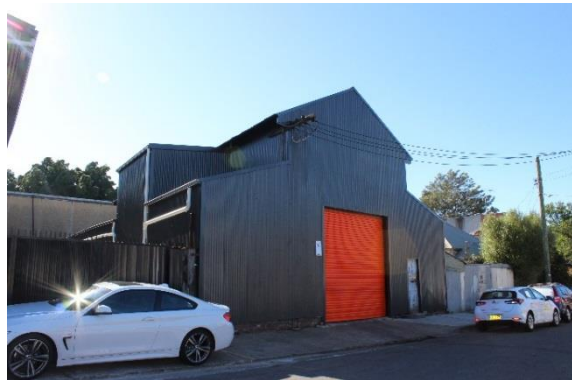
Figure 67: View of front of building, north east aspect
