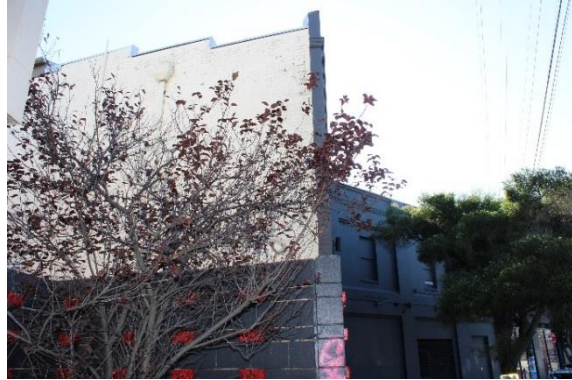
Figure 69: View of side of building, north aspect
