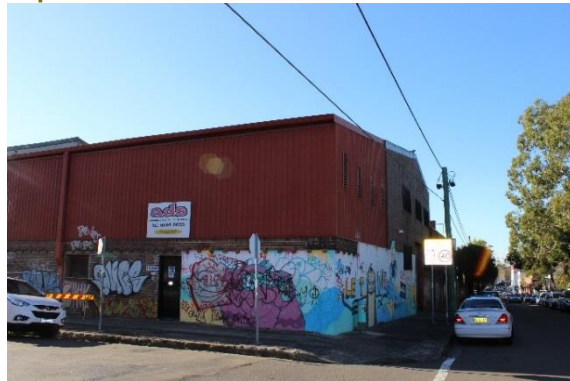
Figure 16: View of corner of building, east aspect
