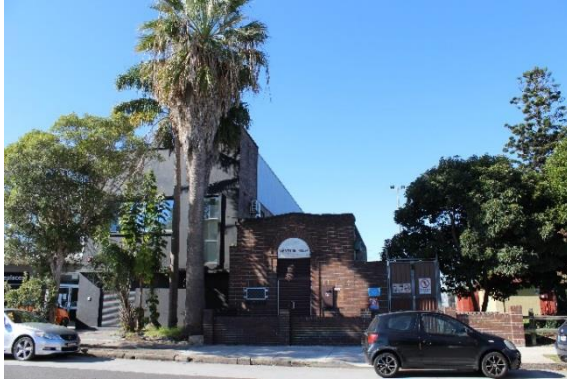
Figure 21: View of building and palm, east aspect
