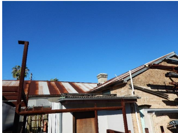
Figure 45: View of original door at rear of cottage 177
