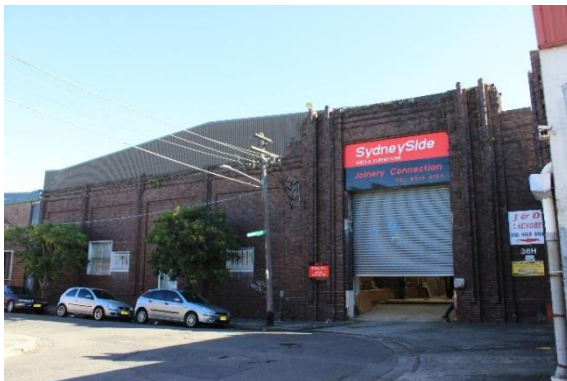
Figure 25: View of façade on Faversham Street, north west aspect
