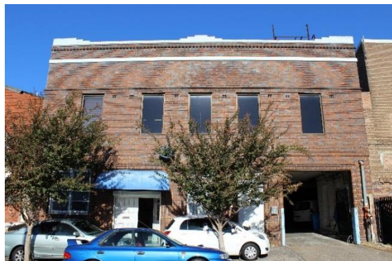
Figure 33: View of No. 14, south aspect
